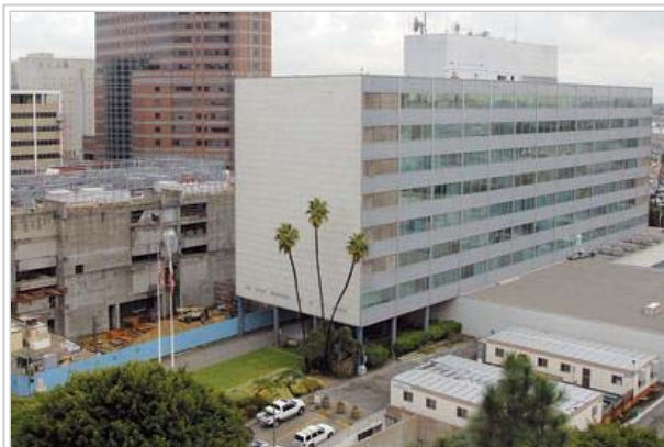
Parker Center, which the LAPD is vacating for a new headquarters a block away, has long been considered for demolition. A proposed study could recommend adaptive reuse instead. Photo by Gary Leonard.
