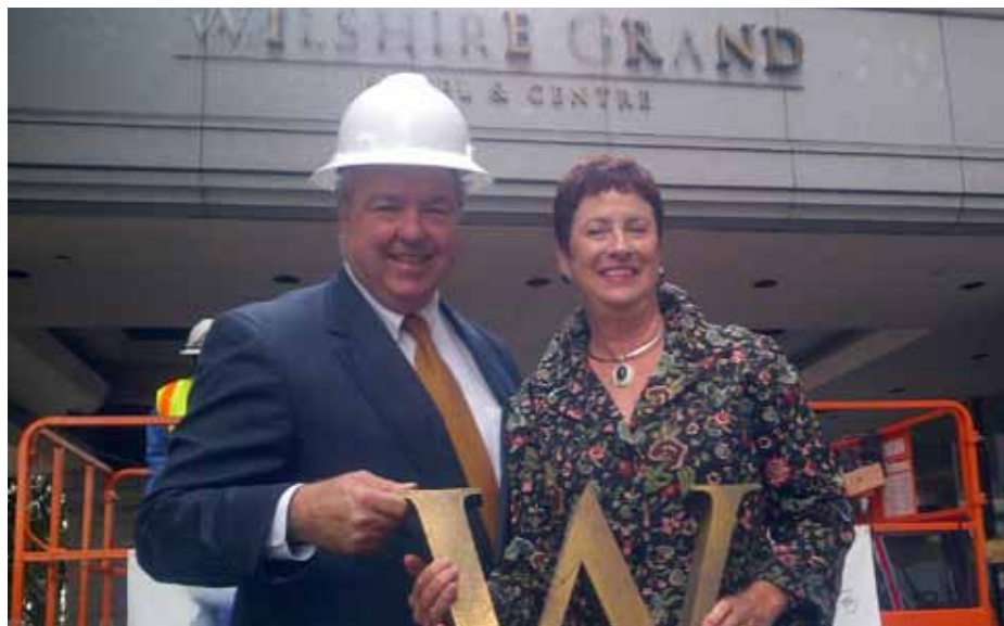
Chris Martin, AC Martin and Martin Project Management and CCA President & CEO Carol Schatz at the Wilshire Grand Hotel demolition
